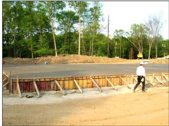
*Fuel from Indian Point's spent fuel storage pools will be loaded into shielded casks and placed on this storage pad. The picture shows the pad under construction.*
