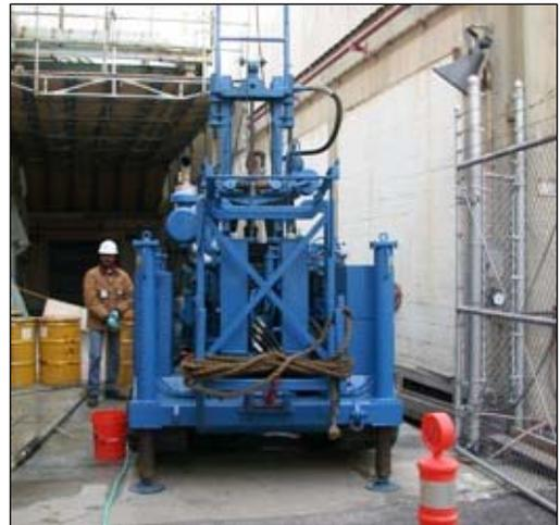
*Drill used to install monitoring wells at Indian Point. Ground penetrating radar is used to ensure that the drill will not intercept buried service lines. Then a vacuum drill is used for the first 6-8 feet followed by a diamond bit drill for the deeper depths.*
